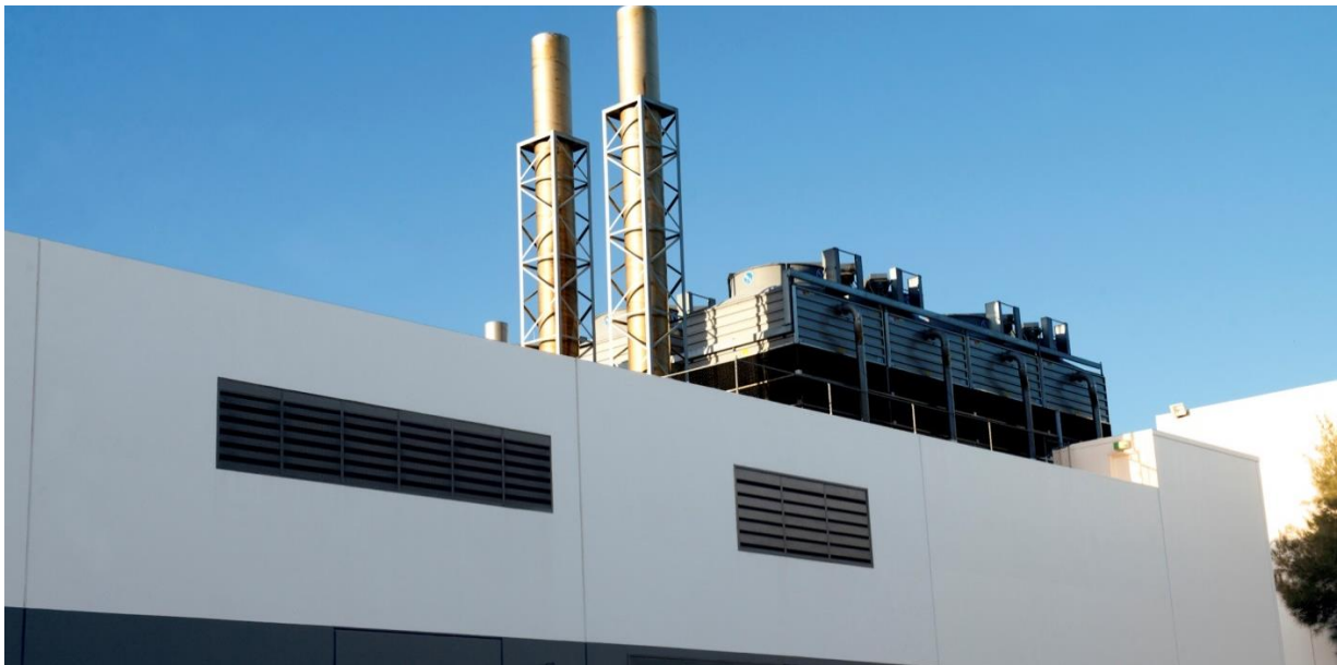
Figure 2 Qantas Jetbase Plant room
